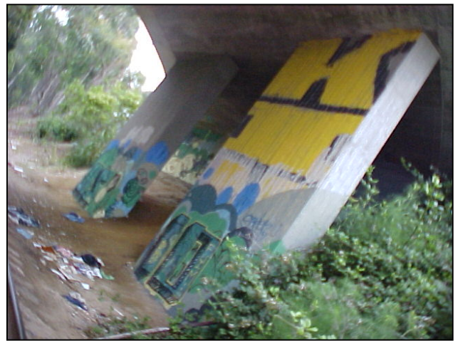
Abutment 1 Looking D/S
