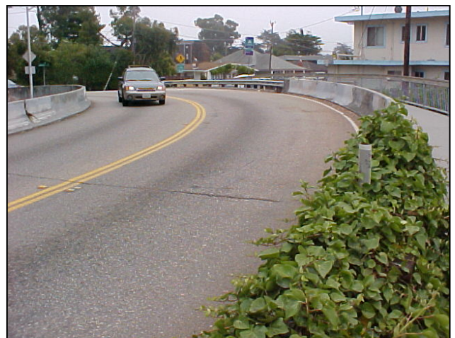
Top of Bridge
