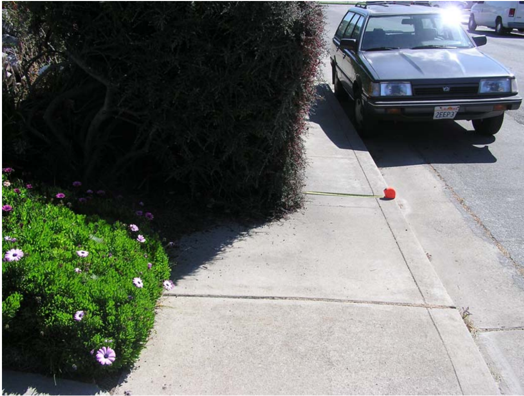
Figure 3. Plant obstructing the sidewalk - before.
