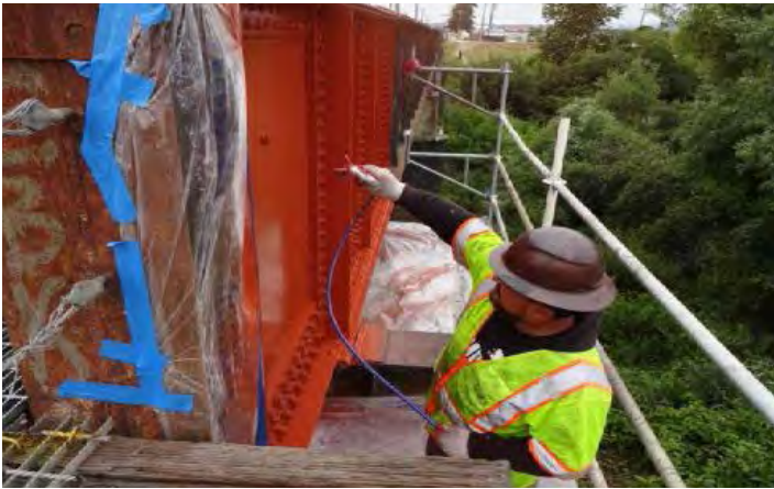
Crews reinforced and repainted the Pajaro River Bridge structural steel.
