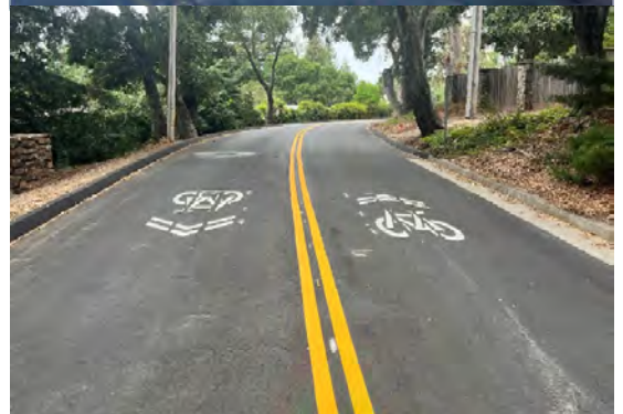
Pavement rehabilitation on Bean Creek Road (before & after), City of Scotts Valley
