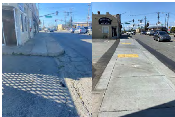
Left: sidewalk replacement (before & after), City of Watsonville
