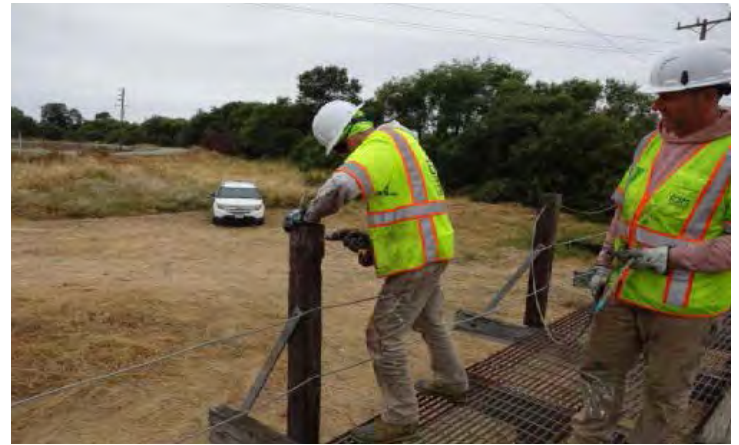
Crews repaired the Pajaro River Bridge cable railing.
