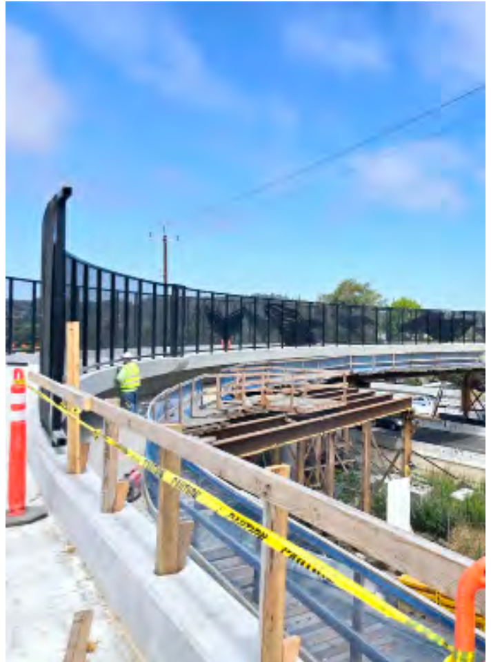
Construction of a new bicycle/pedestrian bridge over Highway 1 at Chanticleer Avenue
