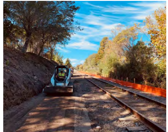
Segment 7, Phase II construction, City of Santa Cruz.
