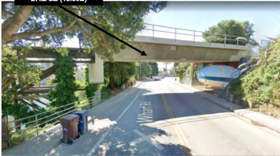
Span is supported by short concrete column bent and abutment
