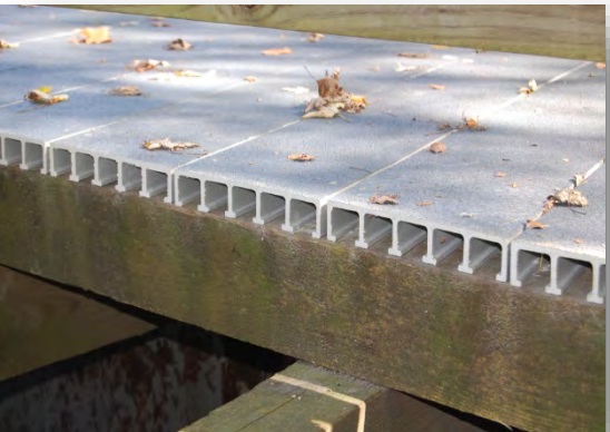
FRP panels installed on truss and timber bridges
