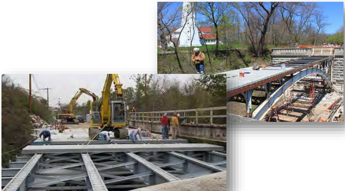
Installation of precast concrete deck panels
