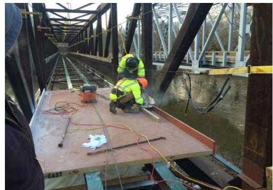
FRP panels installed on truss and timber bridges
