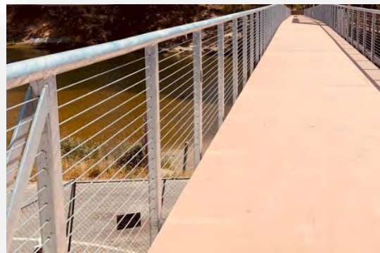
Open metal railing for pedestrian and bicycle used on San Lorenzo River truss
