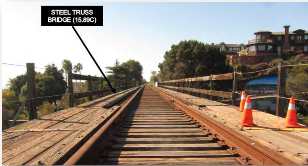
Segment "C" open timber deck for truss
