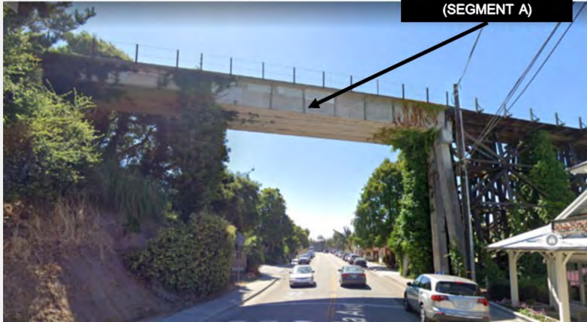
Span is supported by concrete piers
