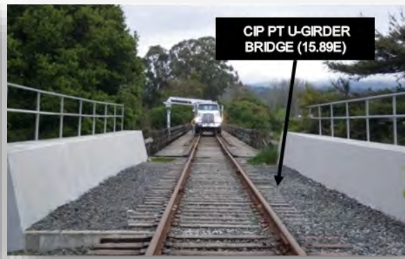
Segments “A” & “E” open concrete decks
