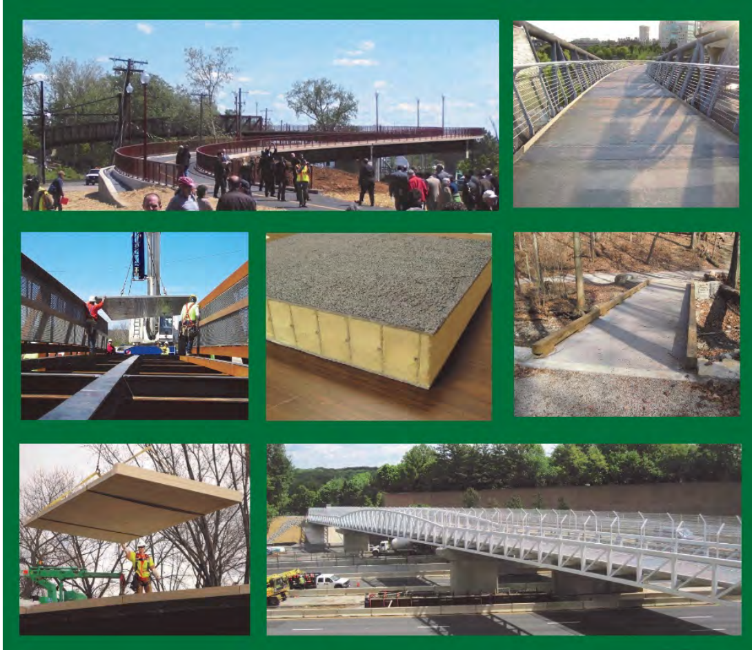
Installation of FRP Panels
