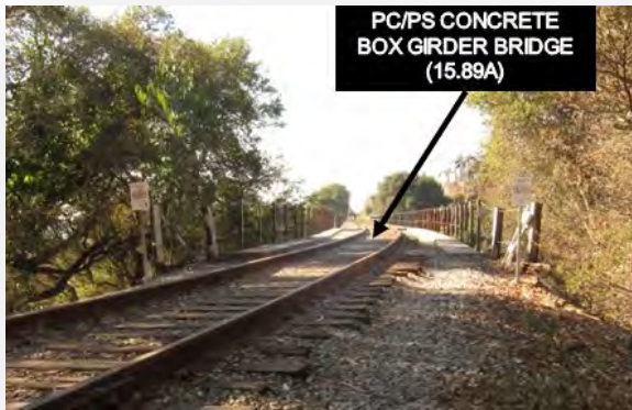
Segments “A” & “E” open concrete decks
