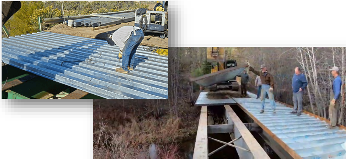
Corrugated steel plank installed over steel girder
