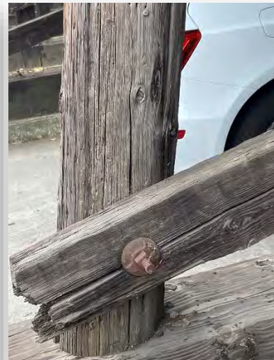
Split bracing at post on mud
