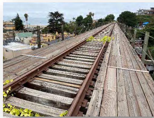
Segment “B” open timber deck
