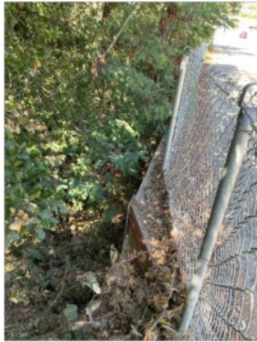
Figure 2 Retaining Wall Failure
