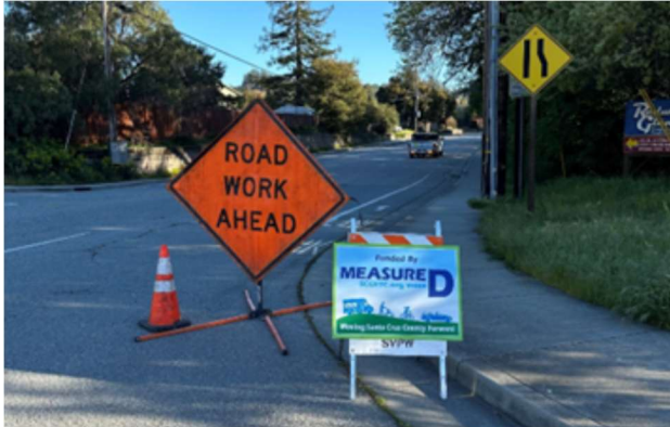
Work on Glenwood Drive
