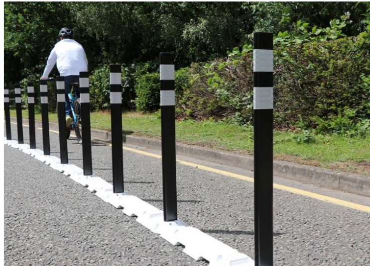
Delineators on Plastic Curb
