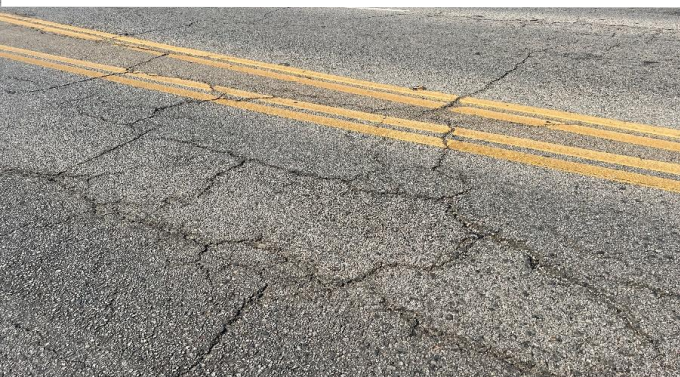
Alligator Cracking
