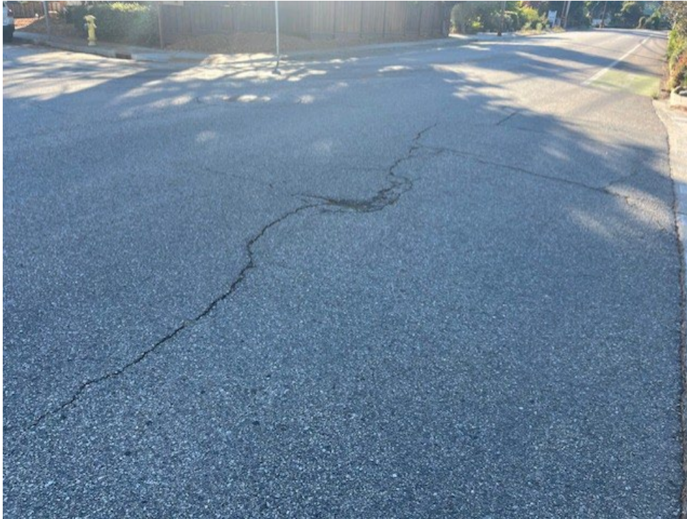
Figure 2 Existing condition on Bay Street at Anthony Street
