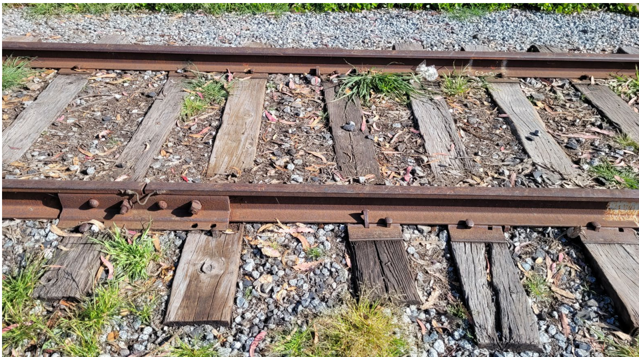
Figure 5.4 Representative Track Structure on SCBRL
