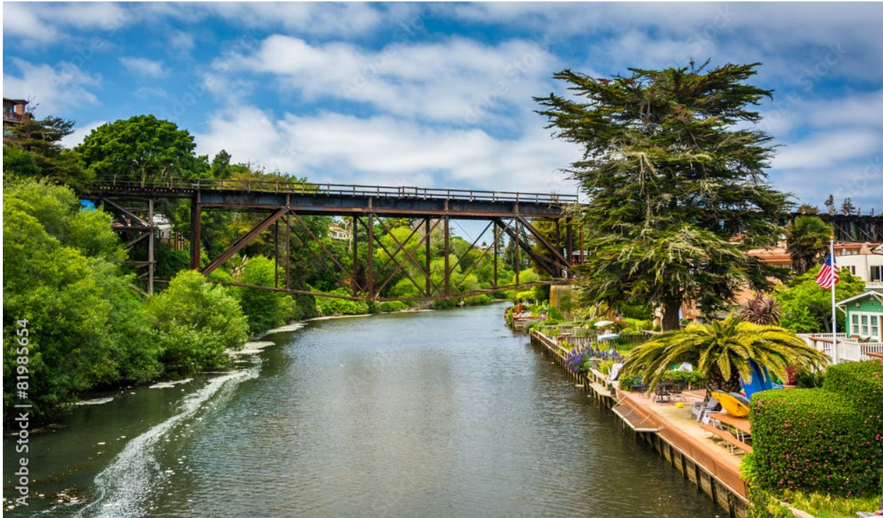
Figure 5.5 Steel Truss Bridge at Soquel Creek in Capitola (Milepost 15.89) on the SCBRL
