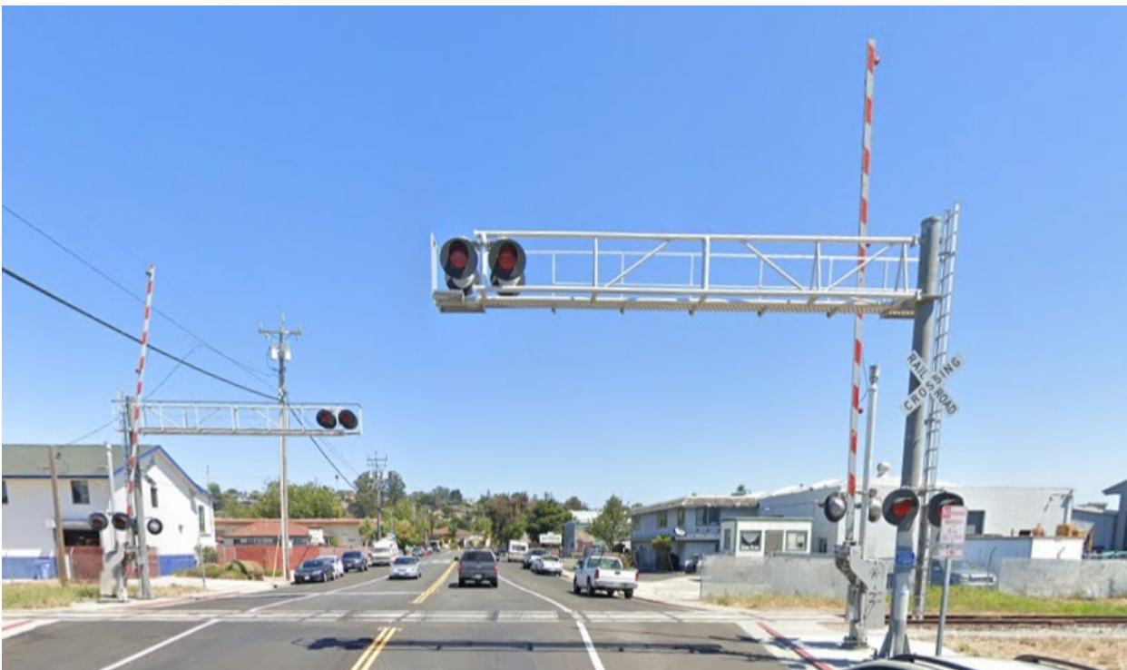
Figure 7.5 Example of Newer Cantilever for Grade Crossing Flashing Light Signals and Signage at Fair Avenue in Santa Cruz (SCBRL Milepost 21.43)
