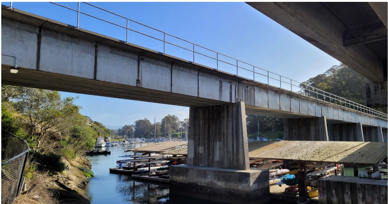
Figure 5.6 Concrete Box Girder Type Bridge at Woods Lagoon (Milepost 18.84) on the SCBRL
