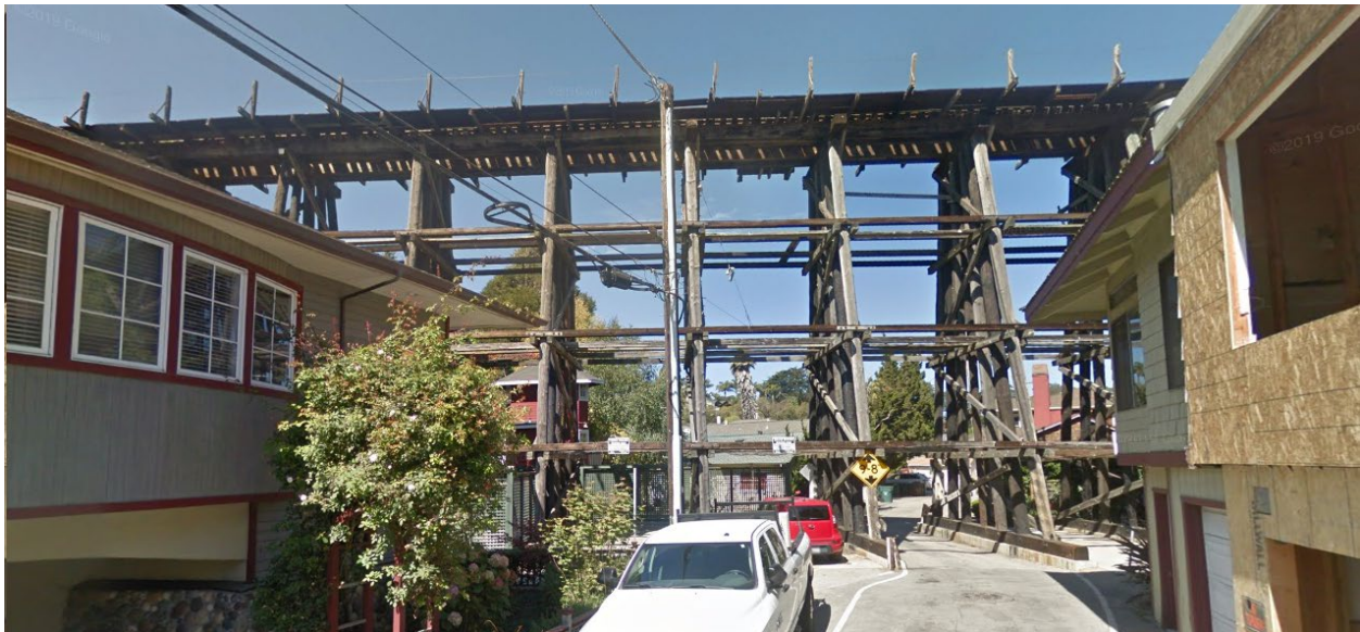
Figure 5.8 Timber Trestle Type Bridge at Riverside Avenue in Capitola (Milepost 15.74) on SCBRL
