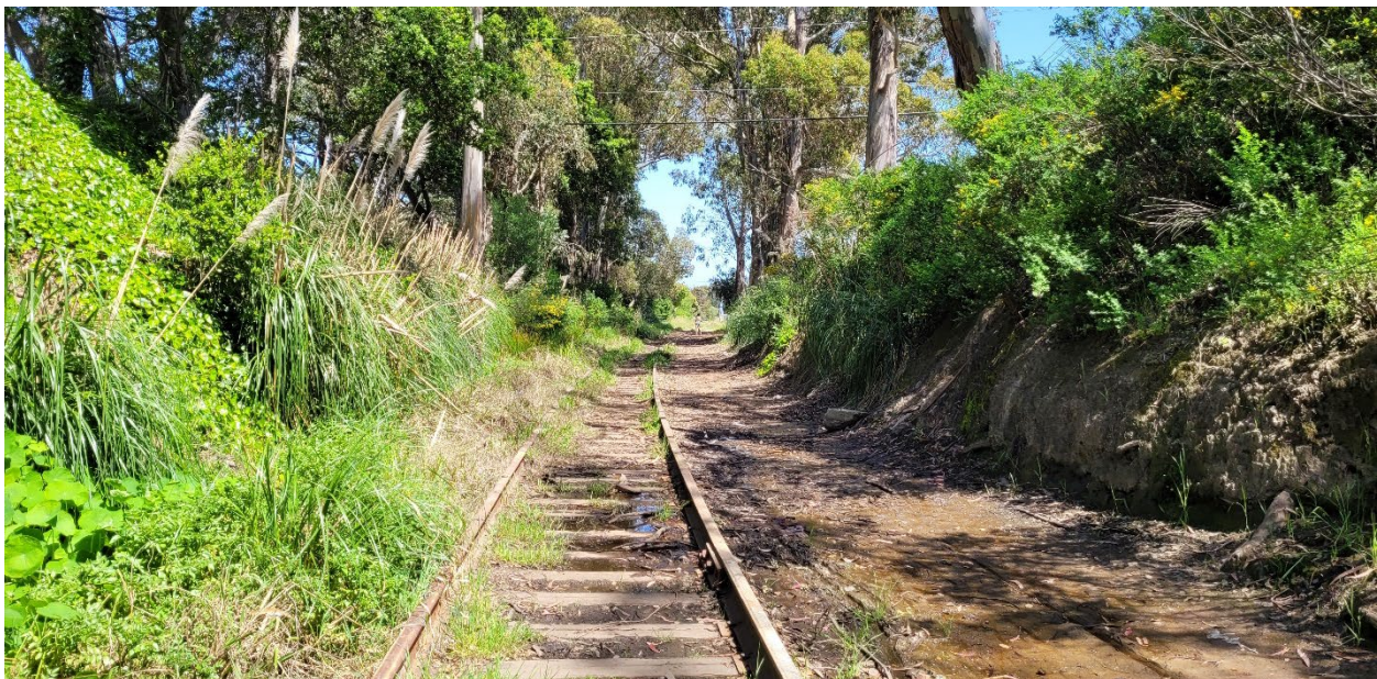
Figure 7.2 Existing Overgrown Track Conditions East of the San Lorenzo River Bridge in Santa Cruz
