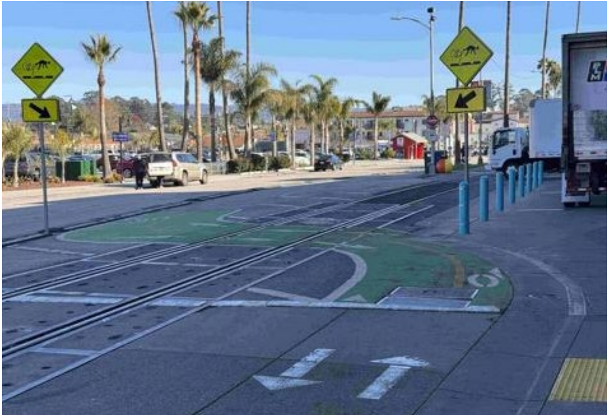
Figure 7.6 Example of Private Crossing at the Beach Boardwalk in Santa Cruz (SCBRL Milepost 19.68)
