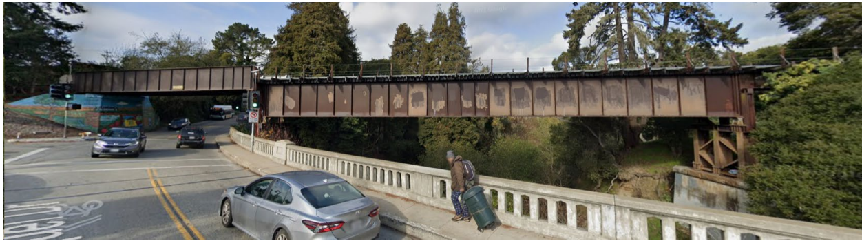
Figure 5.7 Steel Girder Type Bridge at Aptos Creek and Soquel Drive (Milepost 12.71) on SCBRL
