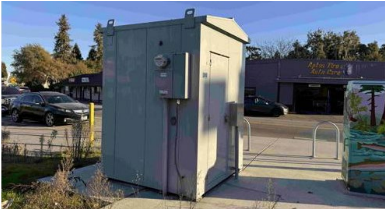
Figure 7.4 Example of Newer Grade Crossing Equipment Bungalow at Aptos Creek (SCBRL Milepost 12.63)
