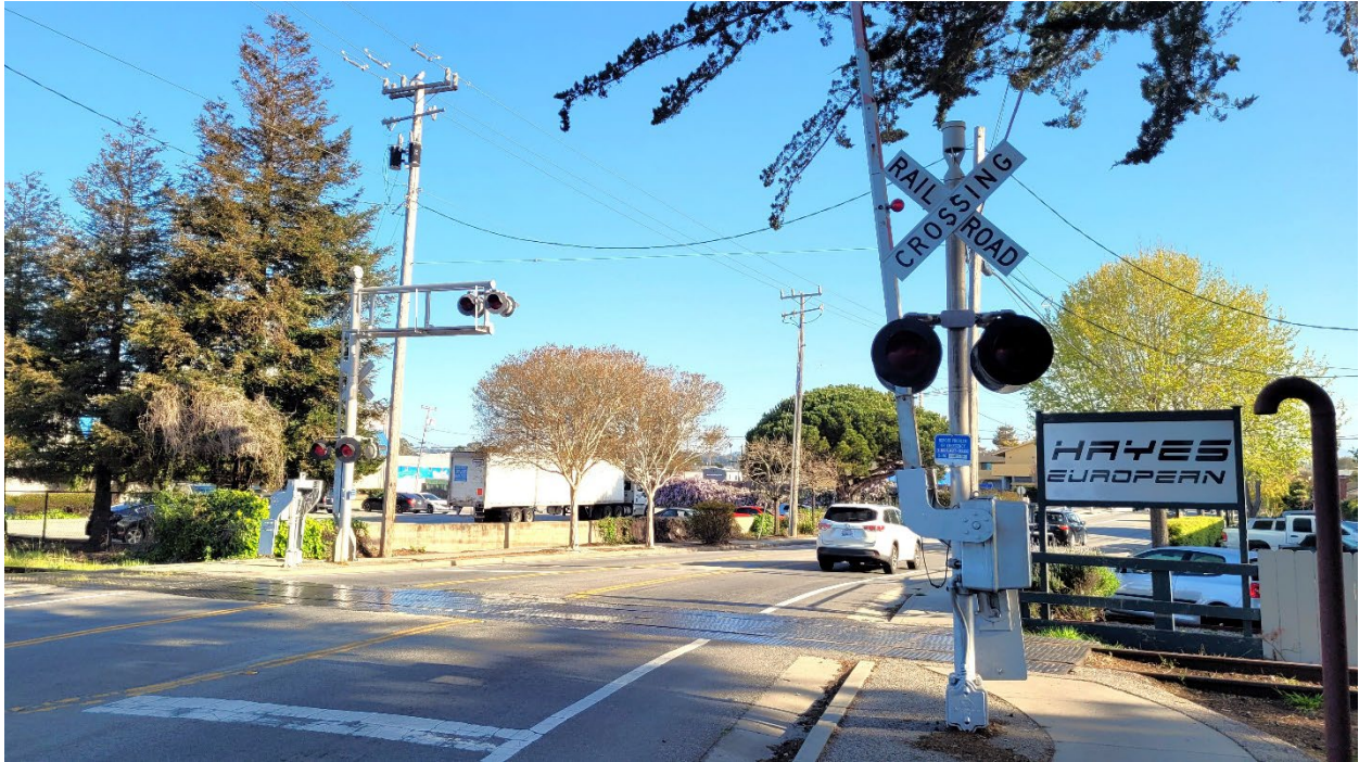
Figure 5.9 Representative Public At-Grade Roadway Crossing with Active Warning Devices at 17th Avenue in Santa Cruz (Milepost 17.83)
