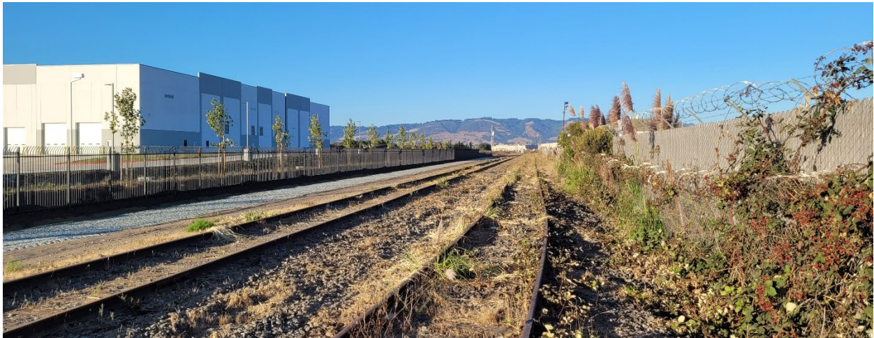
Figure 7.1 Existing Track Conditions in Watsonville
