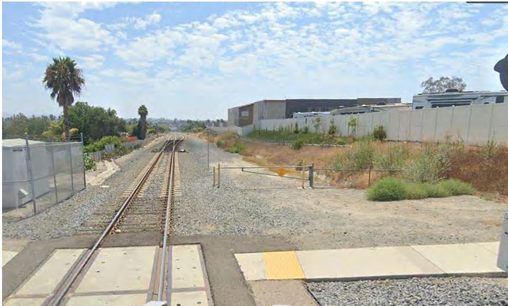
Example of wide and flat right of way along SPRINT corridor at North Drive crossing. Corridor is 100 feet wide, with ample space for construction activities and infrastructure. Photo from Google Earth.
