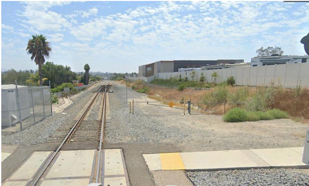
Example of wide and flat right of way along SPRINTER corridor at North Drive crossing. Corridor is 100 feet wide, with ample space for construction activities and infrastructure. Photo from Google Earth.
