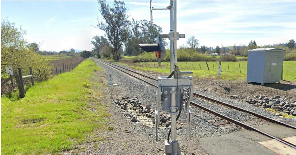
Example of relatively flat right of way along SMART corridor at East Railroad Avenue crossing. Corridor is relatively flat and approximately 60 feet wide. Photo from Google Earth
