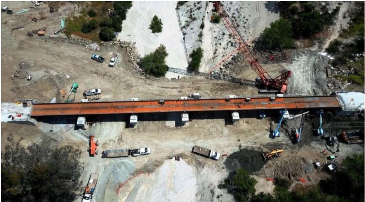
Photo illustrating construction work for replacement of the Santa Ana River bridge for the SBCTA Arrow project and laydown area for equipment and materials on both sides of the bridge. Photo from SBCTA website.
