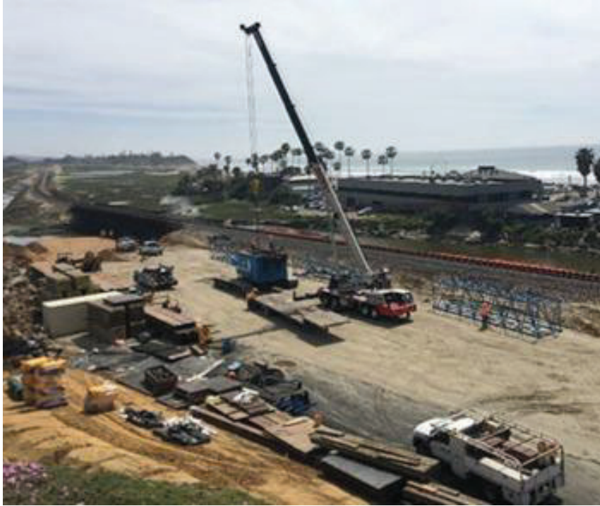
Photo illustrating construction work for replacement of an existing railroad timber trestle at San Elijo Lagoon in San Diego County. Note that at San Elijo, the new bridge was wide enough for two tracks (rather than the single track used for most bridge on the SCBRL) and was constructed adjacent to the existing track in order to maintain that track in operation. Conversely, the ZEPRT bridges would typically be only one track wide and would be constructed on the existing track alignment. However, the width of the freshly-graded area the contractor is using for a laydown pad, materials storage area, and crane work area is indicative of the space needed for bridge construction. Photo from SANDAG website.
