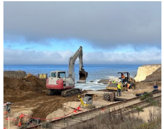
Coastal Rail Trail Segment 5 construction, North Coast
