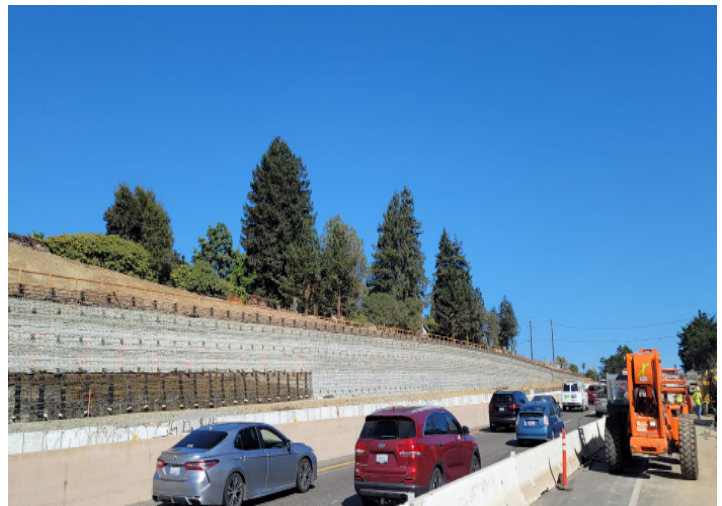
Highway 1 auxiliary lane and bus-on-shoulder construction, Bay/Porter to State Park
