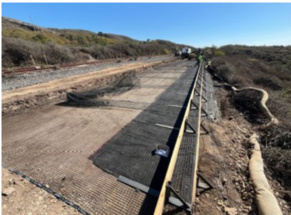
Coastal Rail Trail Segment 5 construction, North Coast
