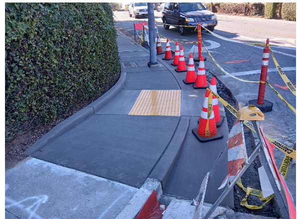
ADA curb ramp construction, City of Capitola
