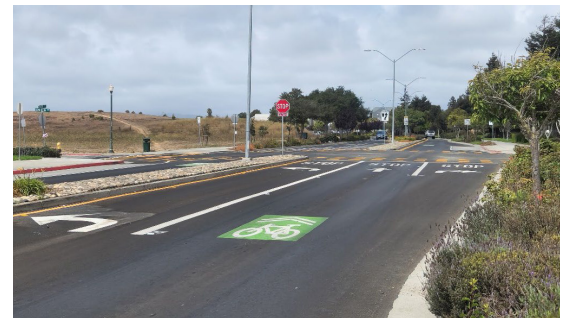
Pedestrian traffic safety improvements, City of Watsonville
