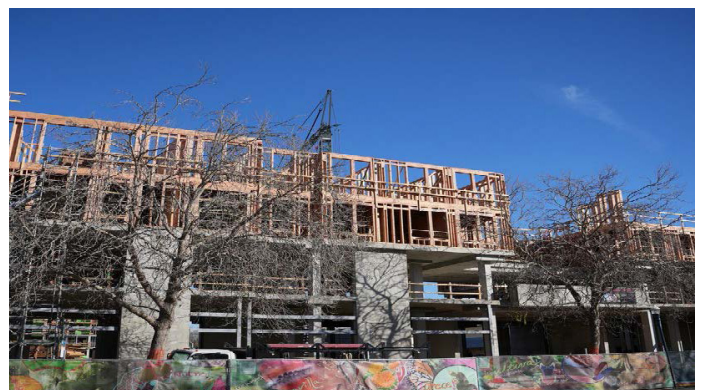
Pacific Station/METRO Transit Center construction
