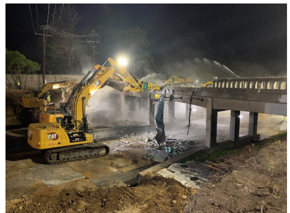
Demolition of the Capitola Avenue overcrossing
