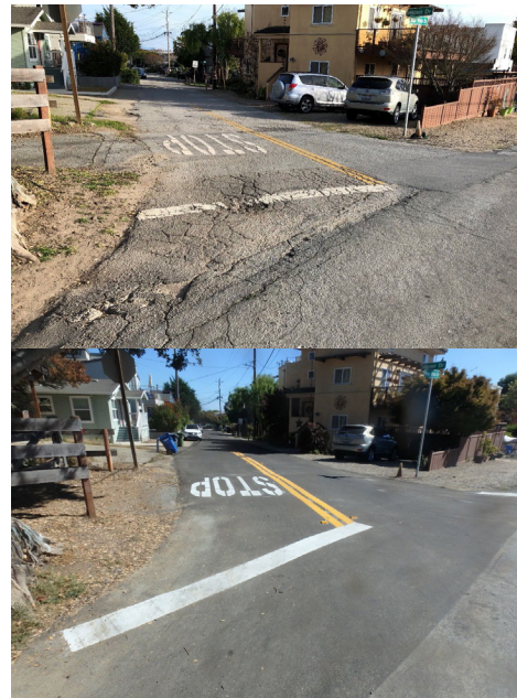
Pavement rehabilitation on Hillcrest Drive (before & after), County of Santa Cruz
