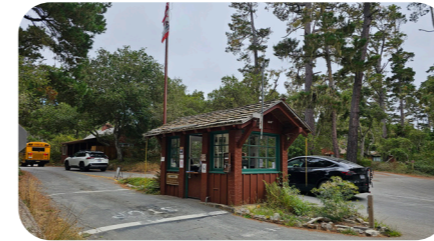
Photo 10. Paid Parking Kiosk - Point Lobos, CA
