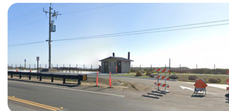
Photo 8. Yellowbank Parking - Santa Cruz County, CA
