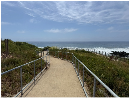
Figure 3. Stabilized decomposed granite coastal access ramp at Tunitas Creek
