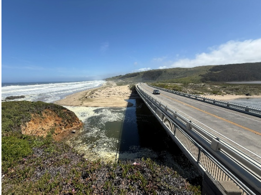
Figure 6. Pescadero Creek bridge
