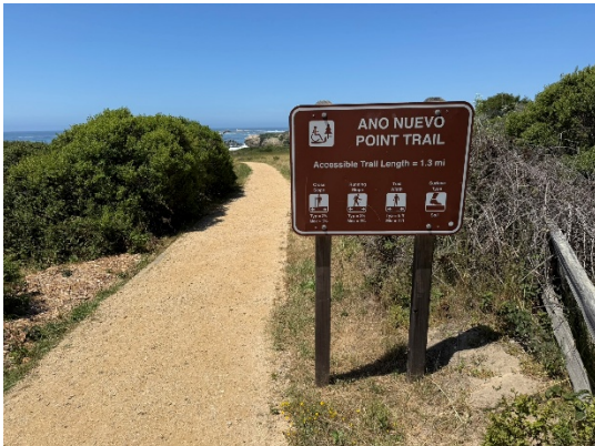
Figure 5. Outdoor accessible crushed rock trail at Año Nuevo State Park
