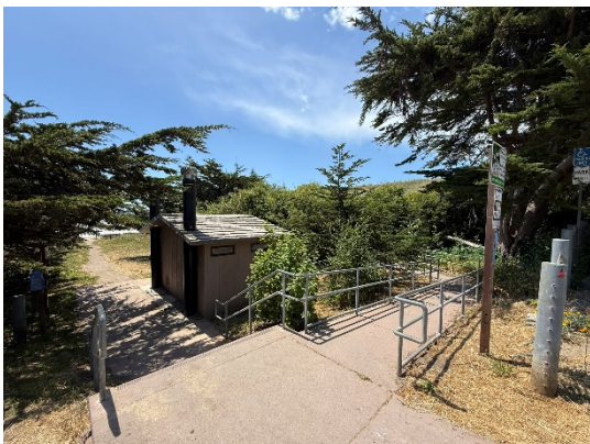
Figure 2. Top of concrete ramp at Davenport Landing
