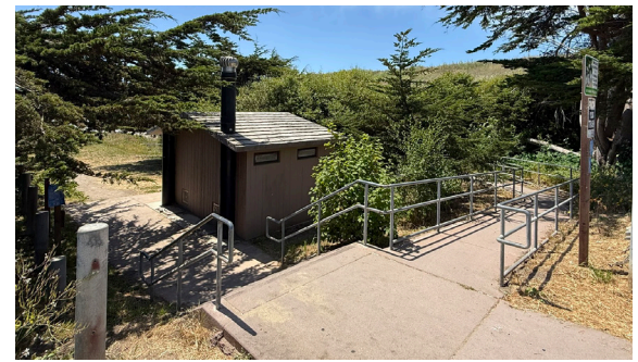
Top of concrete ramp at Davenport Landing
