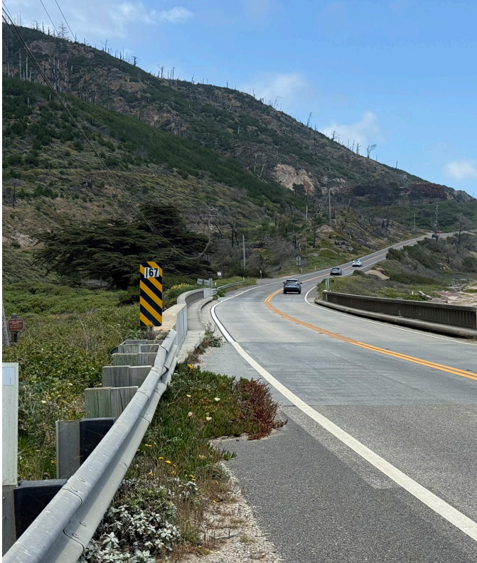
Current Highway 1 bridge conditions at Waddell Creek
