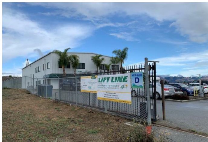
Lift Line facility in Watsonville
