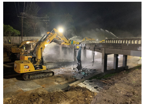
Demolition of the Capitola Avenue overcrossing
