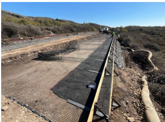
Coastal Rail Trail Segment 5 construction, North Coast
