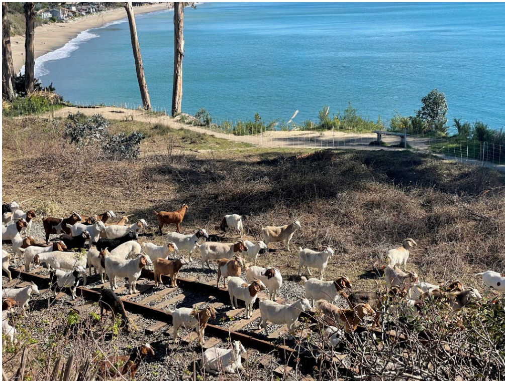
Goat Maintenance on rail line.
