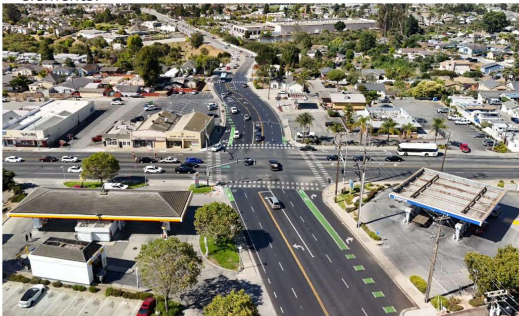
Green Valley Road Reconstruction
