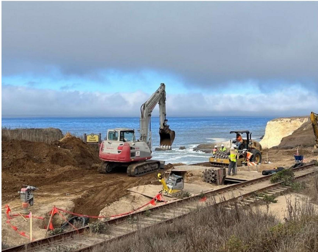
Segment 5 construction, October 2024
