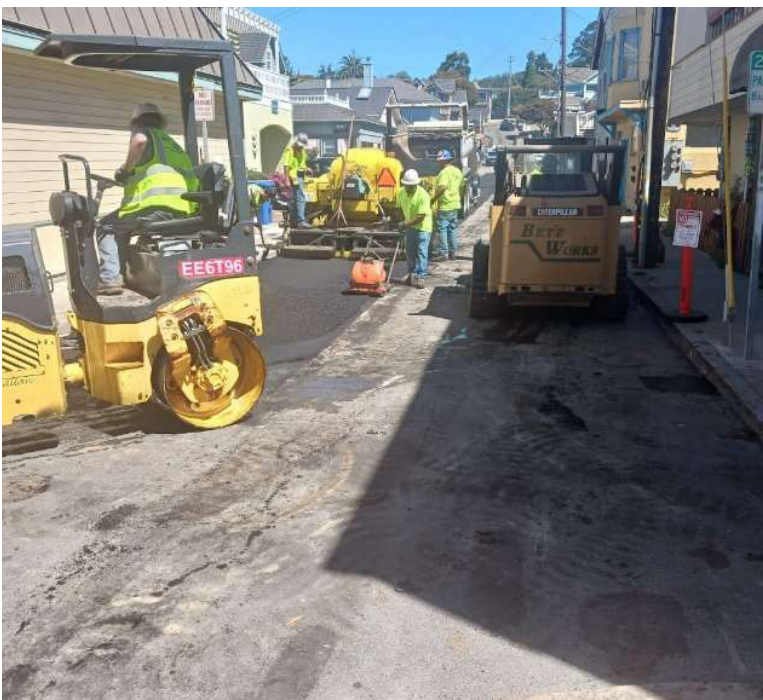
Construction on San Jose Avenue, City of Capitola
