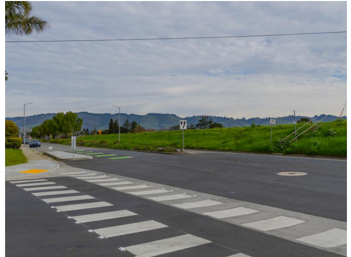
Road resurfacing, City of Watsonville
