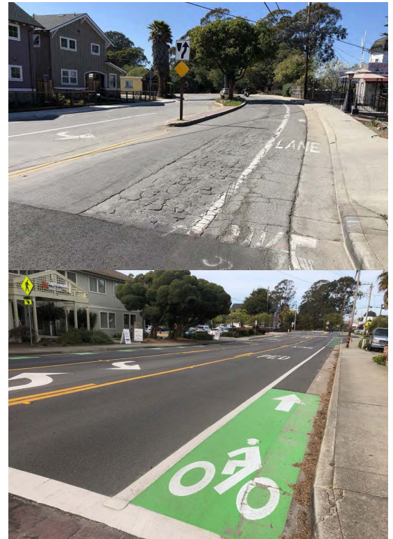
Pavement resurfacing on East Cliff Drive (before & after), County of Santa Cruz
