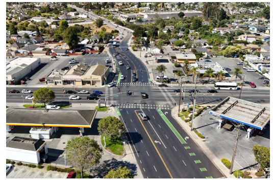
Green Valley Road improvements, City of Watsonville
