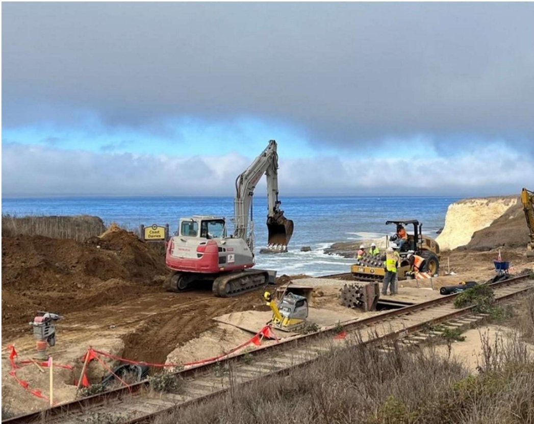
Segment 5 construction, October 2024
