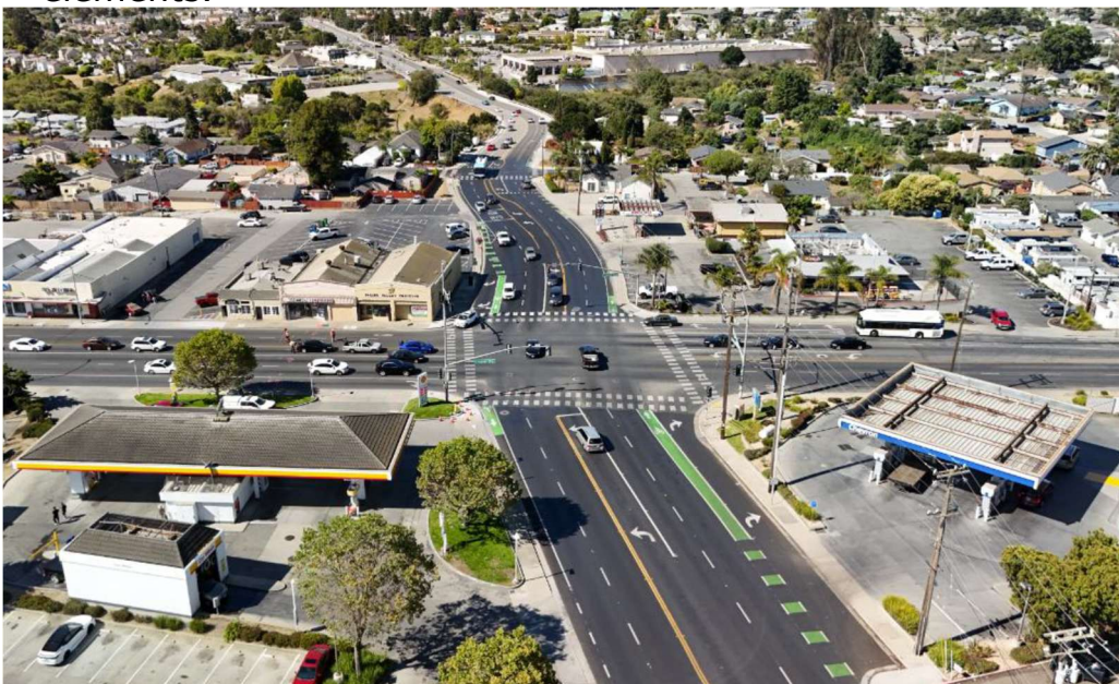
Green Valley Road Reconstruction
