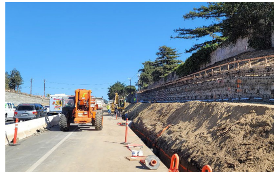
Highway 1 Bay/Porter to State Park project construction
