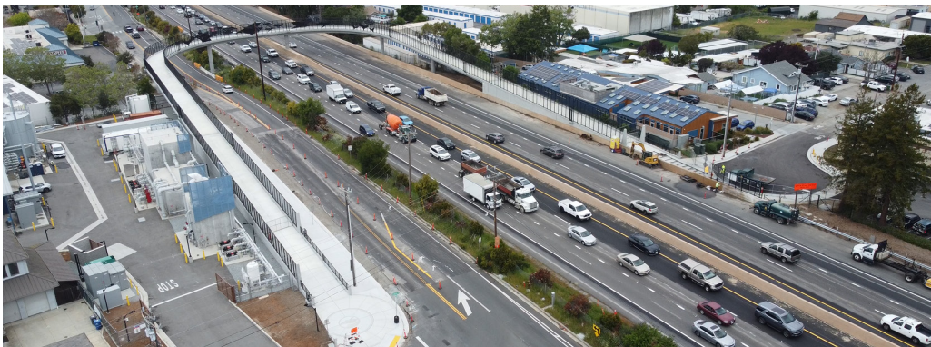
Highway 1 Soquel Drive to 41st Avenue improvements
