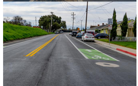
Bridge Street reconstruction (before & after), City of Watsonville
