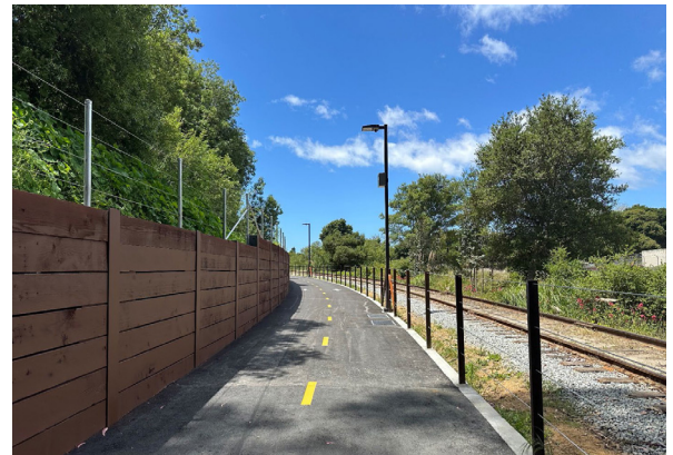
Monterey Bay Sanctuary Scenic Trail Segment 7 Phase 2, City of Santa Cruz
