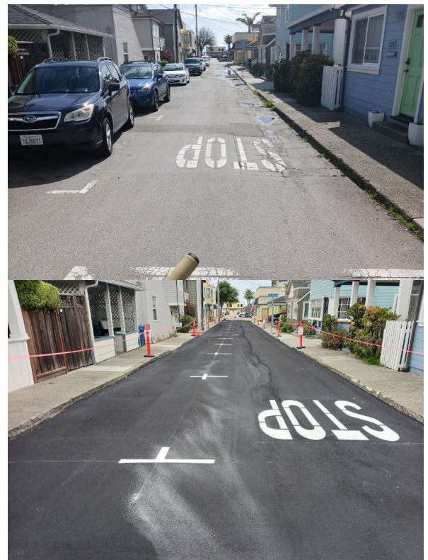
Road treatment on San Jose Avenue (before & after), City of Capitola
