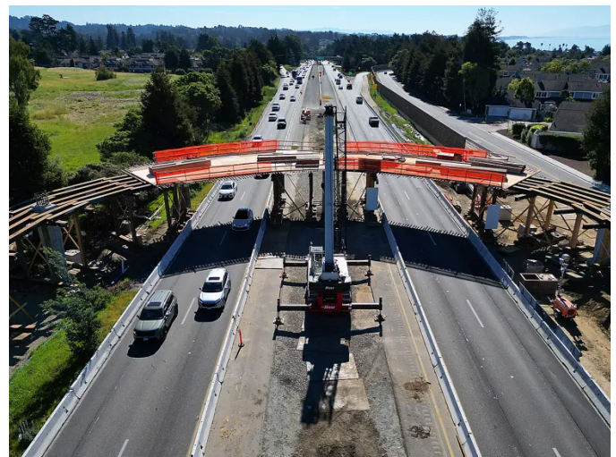
Mar Vista bicycle and pedestrian overcrossing construction, Highway 1 Bay/Porter to State Park project
