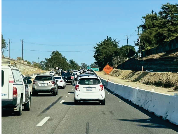
Construction of Highway 1 Bay/Porter to State Park project, October 2024.
