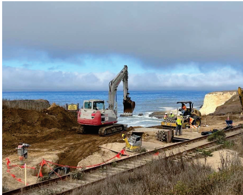
Segment 5 construction, October 2024
